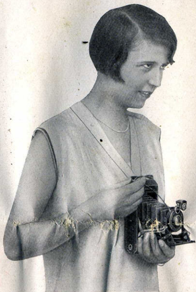
Fig. 4 How to hold the camera for a vertical exposure, when using the brilliant view finder
